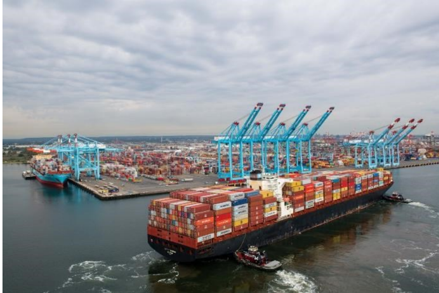
Figure 5.7: Containership at Berth
