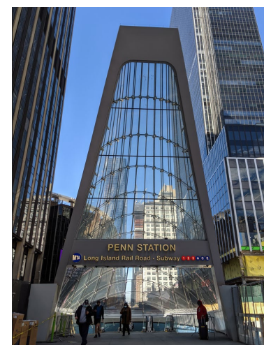
Penn Station Phase 1 & Phase II – New York, NY
