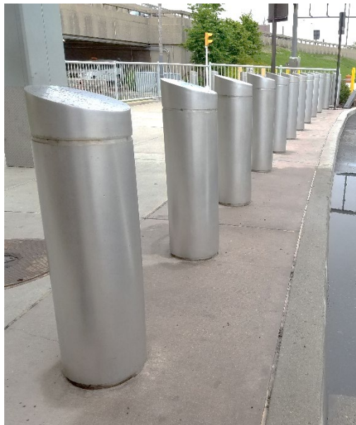
Figure 2 – Security Bollards at Terminal Frontage Roadway
