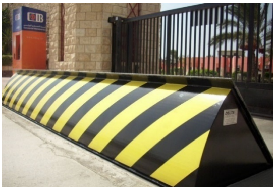
Figure 12 – Permanently Installed Moveable Vehicle Barrier (Delta Barrier or Equal)
