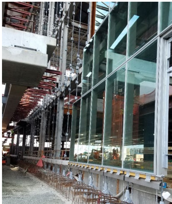
Figure 3 – Blast Resistant Terminal Façade Under Construction
