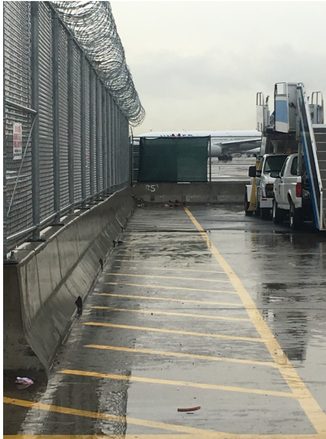
Port Authority AOA Security Fence Requires a Continuous Reinforced Concrete Base Where Any Vehicles May Access the Surrounding Terrain
