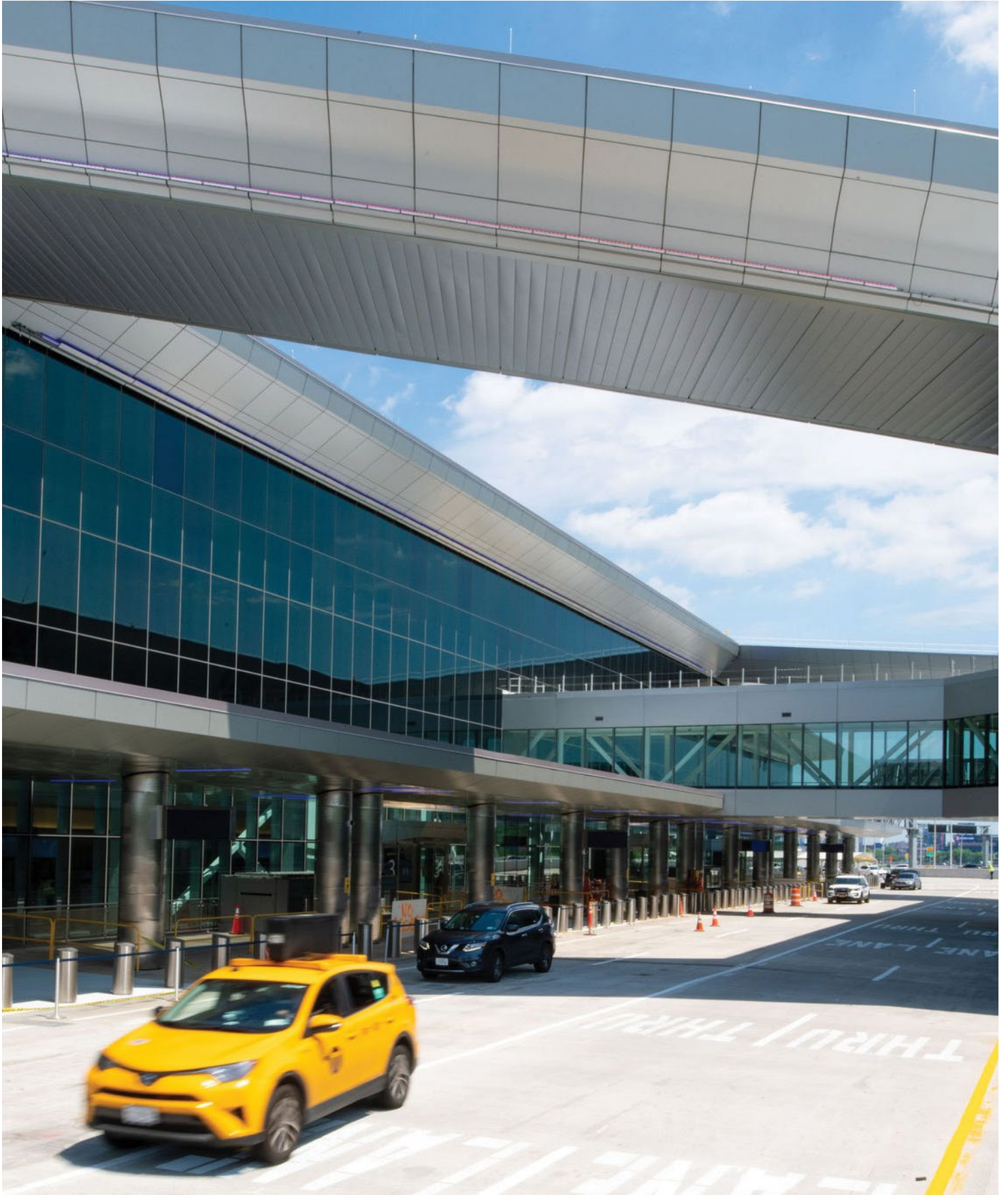
New modern exterior at LaGuardia Airport's Terminal C.
