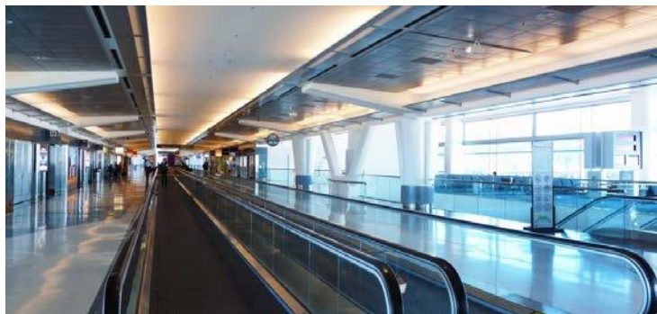
Ceiling height, repetition of structural elements, and lighting design clearly define the passenger flow area.
